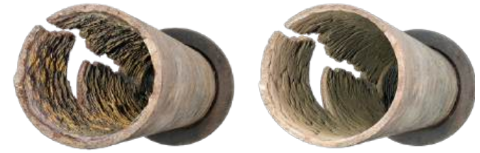
CLEAR ALL BLOCKAGES AND CLEAN THE LINE WALL TO WALL
