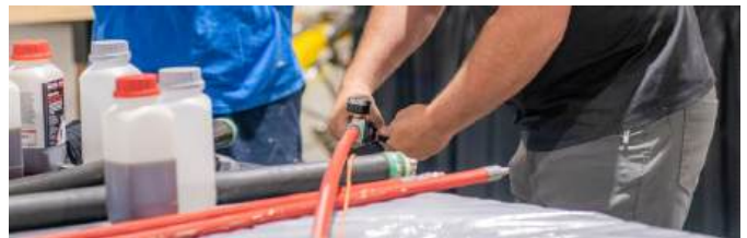
INFLATE THE PACKER TO THE REQUIRED PRESSURE. ALLOW THE RESIN TO CURE FOR THE RESIN SET TIME.
