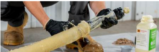
PREPARE THE PATCH AND PLACE THE PACKER AT THE REPAIR POINT.
